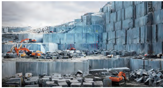
Stone excavation & cutting
